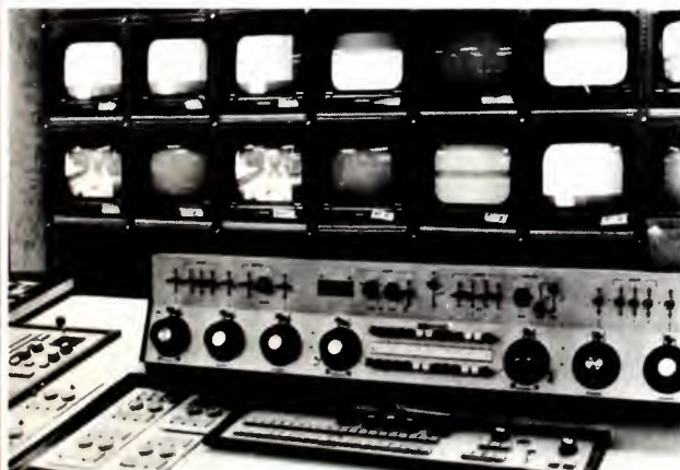
Master control room also serves as Studio A control. Remote switching panel (below Gates audio control) makes it possible to handle Studio A production and on-air signal. CCU, sync generator, DAs, etc., are directly behind switching console.
