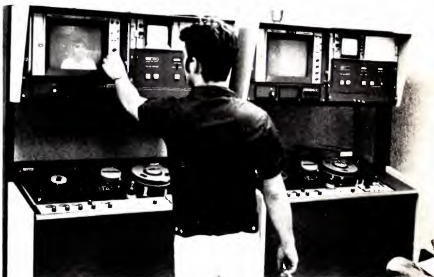
Most all locally produced programs will be played on IVC 960 helical recorders. Two quads are in the same room.
